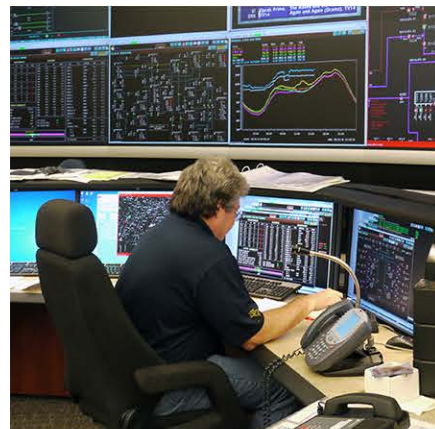
Hawaiian Electric recently upgraded its Energy Management System, the “brain” that controls the electric system.
